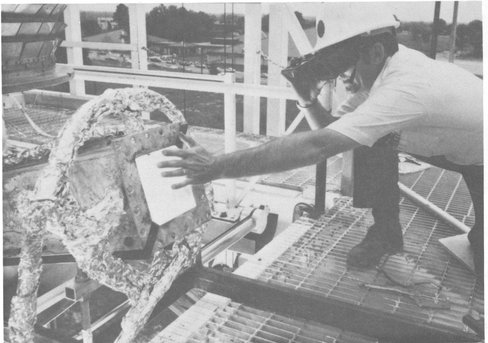
Tom Brown, ERL, perched on a tower 72 feet above the ground, gazes into the eye of a light pipe being tested at the Georgia Tech/Department of Energy solar furnace located on campus. This month the pipe will be further tested at a 1000 kilowatt solar furnace located in Odeillo, France. Steve Bomar and John Handley, both of ERL, will brave peak season skiing crowds in the small Pyrénées town to conduct tests which may lead to more information about the effects of nuclear explosions. Soil samples will be placed inside the pipe and struck with high amounts of solar radiation, simulating the effect of the blast of an atom bomb on the earth's surface.
