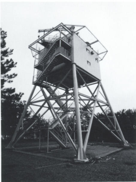
The receive tower can accommodate antennas weighing up to 40,000 pounds.
