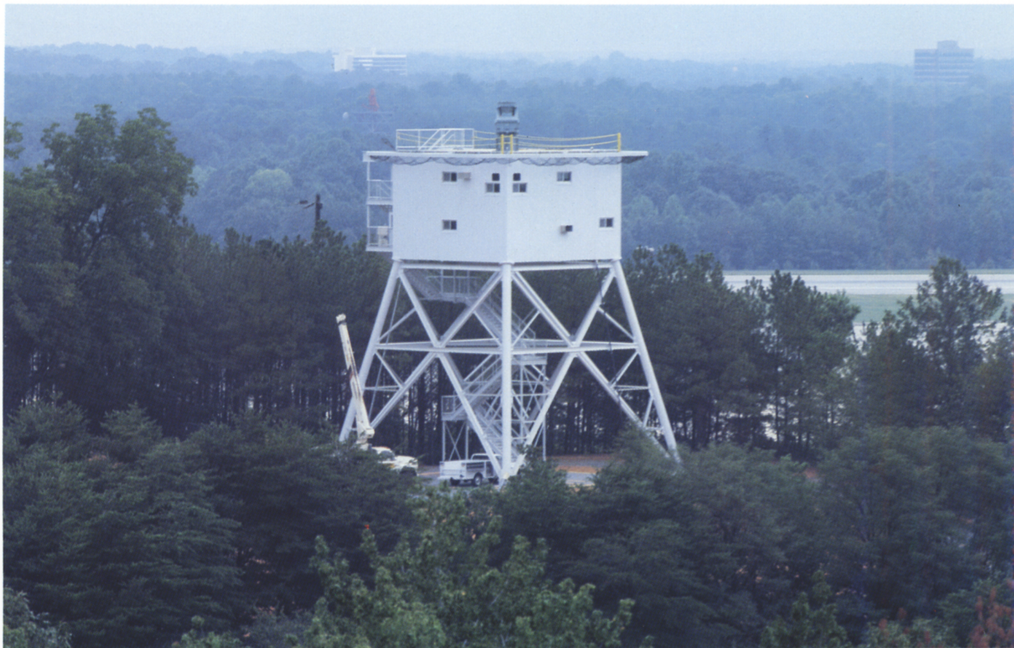
Georgia Tech's Electromagnetic Test Facility is located at the university's Cobb County research complex near Dobbins AFB. Shown here is the far-field antenna range's 64-foot receive tower.
