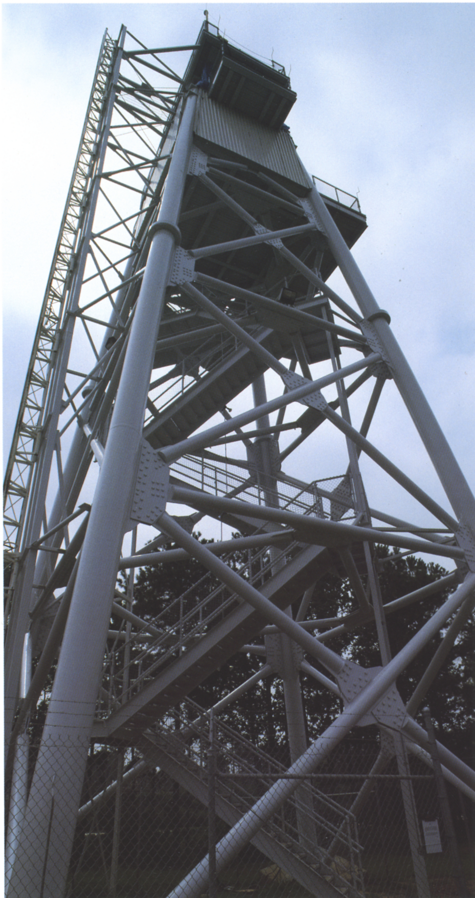
The source tower of the far-field antenna range is stable enough for use in boresight testing of precision tracking radar systems through the millimeter wave region.
