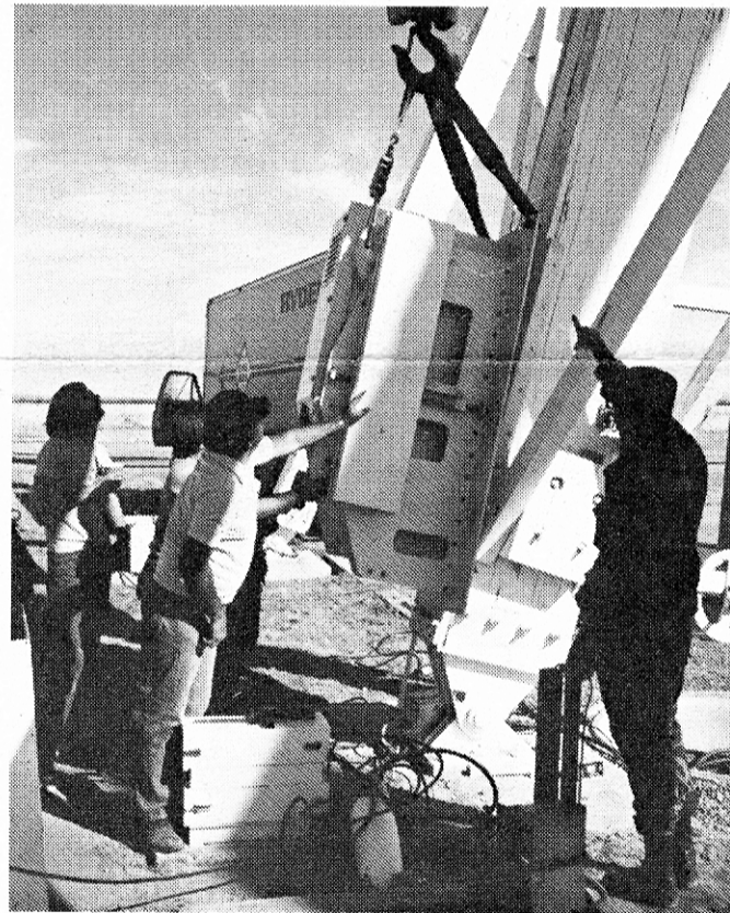
STL engineers designed a new automated antenna testing system for the "arch" range at Fort Huachuca, Arizona (above). The arch has a 75-foot radius and is centered over a turntable. STL developed the software, procured the computers, and equipped the range with new instrumentation. The photo at left shows installation of the drive mechanism. (Photos by Henry Cotten)
