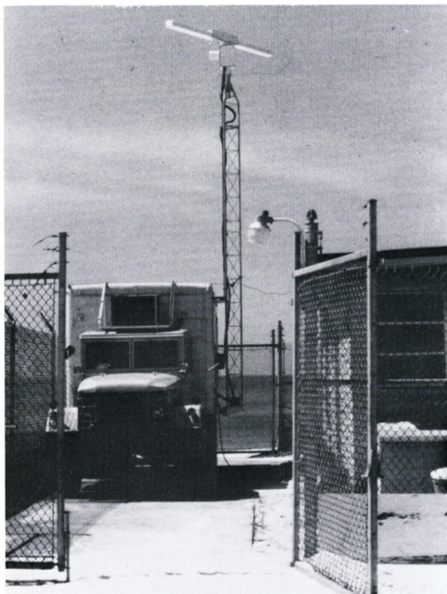
EES-developed radar system at Panama City, Fla., warns against unauthorized waterborne traffic.
