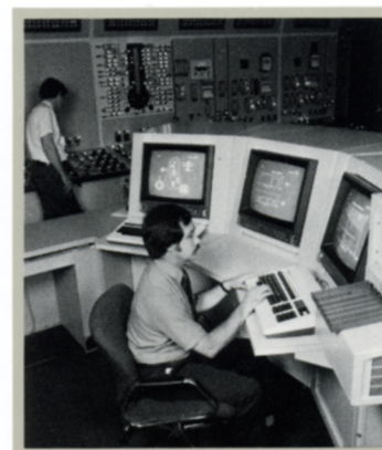
Station engineers installed this simulator of a Safety Parameter Device System at Georgia Power Company's Plant Hatch.
