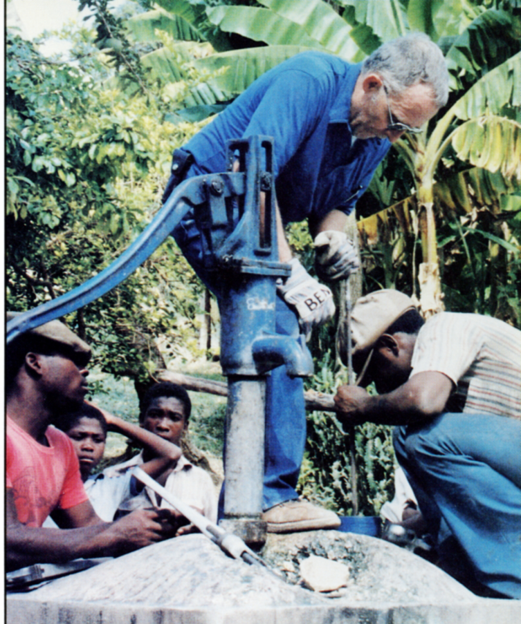
(Left) An EES technical assistance team is helping Egypt to set up an industrial extension program similar to the Station's field office system. (Above) An EES engineer trains Haitians to install the U.S. AID hand pump for safer drinking water.
