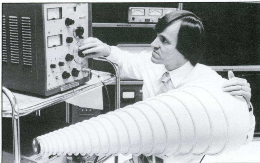
EES electromagnetic compatibility specialists are using this antenna to study radio signal penetration of buildings.
