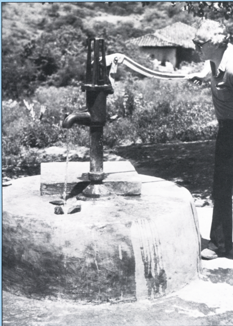
To help underdeveloped countries obtain clean water supplies, EES staff members taught native engineers to install and maintain hand-operated water pumps.
