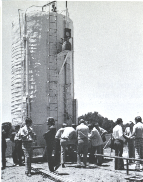
The EES 10,000-gallon anaerobic digestion system converts manure into energy.
