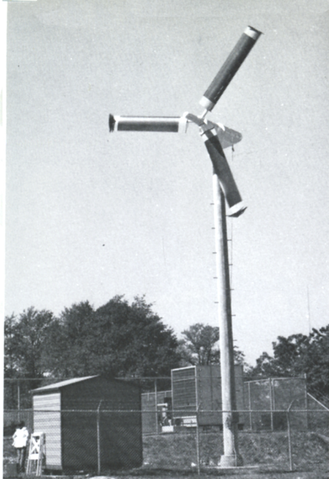
The Georgia Tech 15kW Grumman Wind Generator used in wind energy systems analysis programs.
