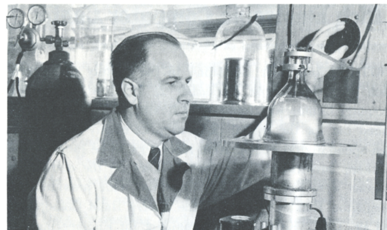
Sputtering system used in Georgia Tech's thin metal research.
